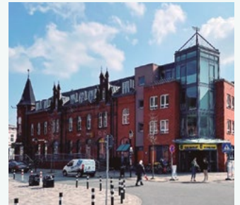
The EDEKA store in Germany, the first supermarket providing the maintenance-free nanoe™ X technology for better indoor air quality. Germany. ECOi and nanoe™ X
