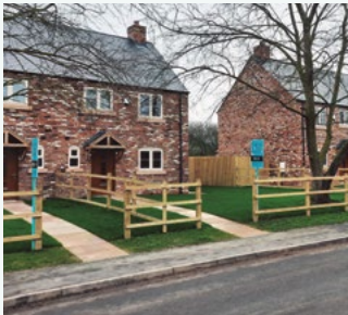
Aquarea Heat Pumps provide heating and hot water for new rural housing development, UK. Aquarea
