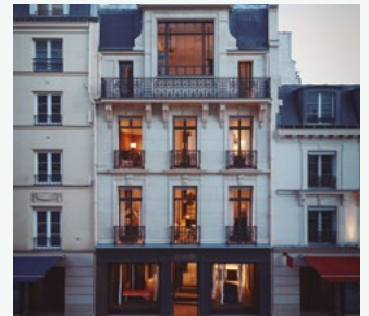
LIAIGRE showroom, well-known as a luxury design architect in Paris, France. ECOi
