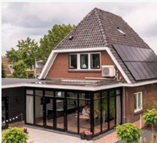
Aquarea T-CAP provides a complete solution of heating, cooling and DHW for the refurbishment of a luxury house in Voorthuizen, Netherlands. Aquarea
