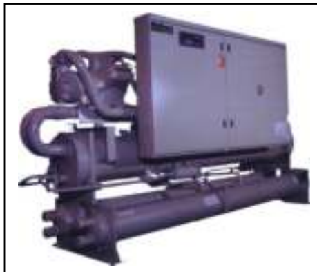
Figure 65 - Templifier™ in a Condenser Loop
