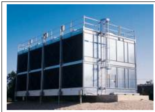
Figure 15 - Induced Draft Cooling Tower
