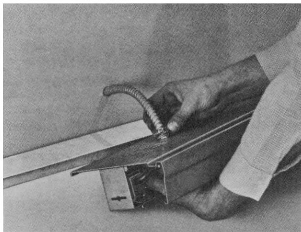
Figure 2-69 Making the electrical connections.
